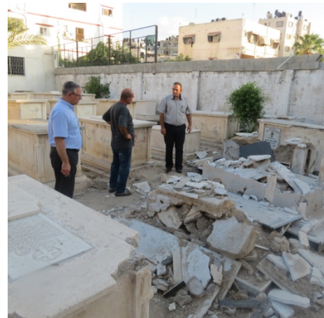
Even cemeteries were not spared! Checking the damages at the Greek Orthodox Church cemetery, Gaza City.
